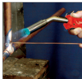
Hardsolderen
